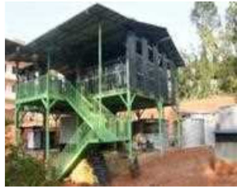
1 MLD STP at Kozhikode medical College
